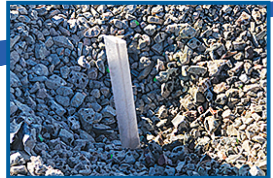
A single wick drain.
